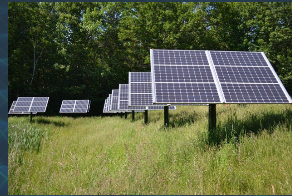
Use of Energy
