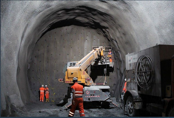
Reuse of excavations
